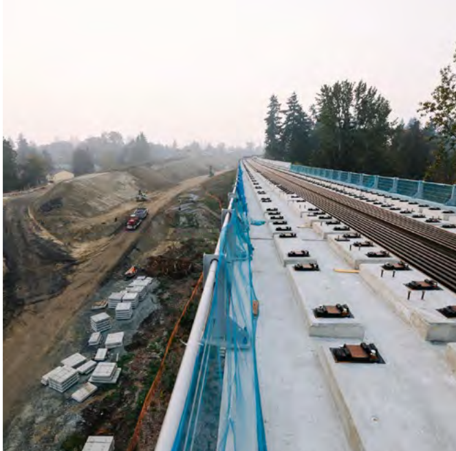
Continuing expansion: Connecting new tracks to our existing network.
